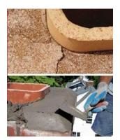
Today we are going to cover repairing the chimney crown. If during the inspection process you notice that the chimney crown is cracked and chipping away this is not a good thing. It should be repaired before the temperatures drop. If water was to get into the cracks and ice over it will just continue to make the cracks worsen or start to break away from the chimney. To repair the chimney crown it will need to be sealed with a waterproof sealant.
