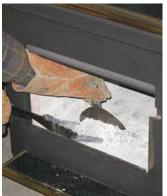
To maintain a healthy wood stove keep the ash build-up in the firebox to a minimum. Make sure that you are emptying the ash drawer or scooping the ashes out daily. There should only be a thin layer of ash in the bottom of the firebox. Having excessive amounts of ash in the firebox will only clog up your stove. You fire will not burn efficiently because it will not be able to get the air circulation that it needs.
