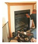
Have your chimney and wood stove(s) cleaned and checked every year. Replace worn gaskets during the warmer months. This will improve the efficiency of your woodstove as well as its safety. Also, check the stove, stovepipe, and chimney flue regularly during the heating season. Consult an expert if you have any uncertainty about how to conduct these checks.
