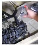
Now place the Lava Rock, a.k.a. Cinders, along the floor of the firebox surrounding the grate. The lava rock is supposed to make the appearance of ash or cinders. Now finish putting down the rest of the rock wool to fill any holes or gaps between the silica sand and lava rock. Make sure that the sand is completely covered. The sand is where the gas comes from and the flames will make the rock wool look like glowing embers. Don't be stingy with it, put it anywhere you can.
