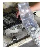
After the grate is in place you will begin to place the rock wool, a.k.a. glowing embers, under the grate starting in the back and working your way to the front. Leave some room in the front so that it does not fall to the firebox floor and get covered by the lava rock. You can use the rock wool to cover the gas fittings so they are hidden. The rock wool will not glow over the fittings as there will be no gas flowing through them but it will keep the fittings from being obviously seen.
