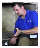
Start by applying the pipe dope or Teflon tape to the connecting end on the burner pan. Be as careful as possible as the pipe dope does not come out of carpet or clothing very easily, if at all. Always use two wrenches when you are working with gas line fittings. You do not want to spin something that is already tightened. This could cause you to create a leak in the line without even realizing it. Make sure that the gas feed will be pointing to the back of the firebox.
