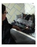
After you have the firebox all set up the way that you like it, it is time to turn on the gas and light the fire. We did not include an ignitor in our installation so we will be lighting our fire with a long stick match. Have the match lit and placed under the grate above the rock wool as you turn the gas on to the fireplace. Once the flame is lights you are all done! Ta-Da! Now all you do is sit back and enjoy the beautiful realistic gas fire!
